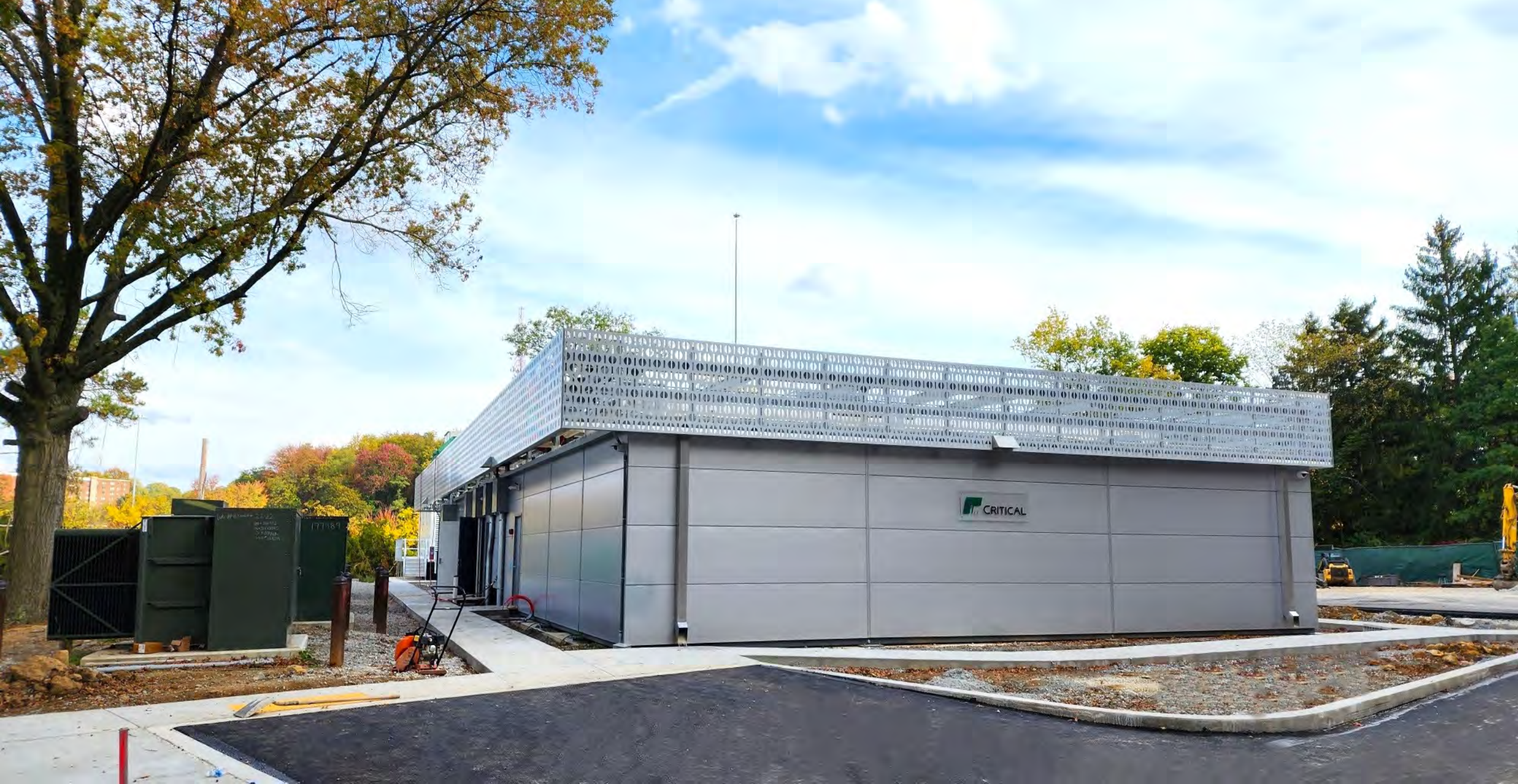
iM Critical Data Center – Pittsburgh, PA (10 modules, same form factor)
