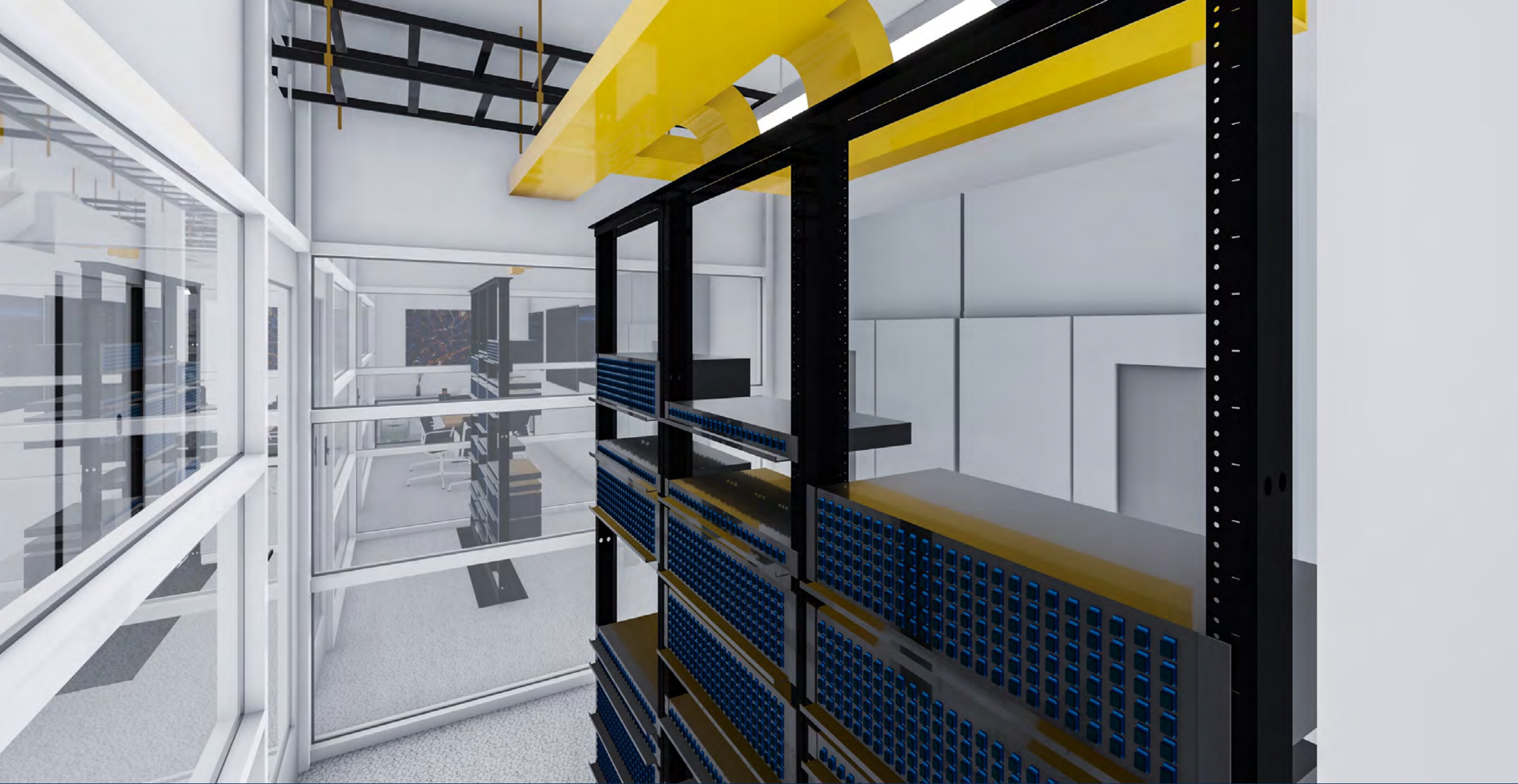
Passive Fiber Distribution Panels in Meet Me Area A (with Meet Me Area B in the background)
